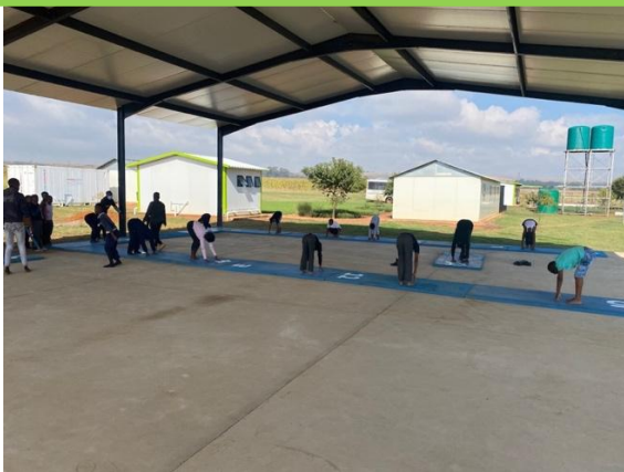
Open Hall Structure
