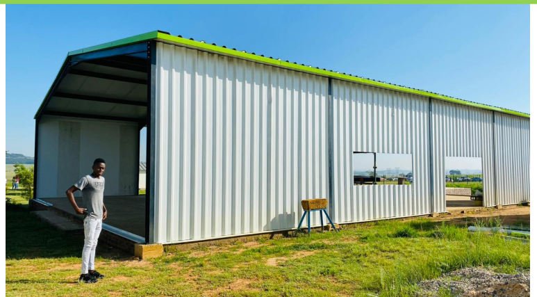
Hall under construction
